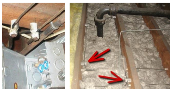
(left): Old and newer wiring often co-exist; (right): Location of the knobs in attic indicated by red arrows.
