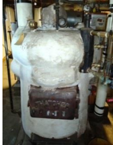
Examples of asbestos insulation wrapping boilers and associated pipe insulation encapsulation.
