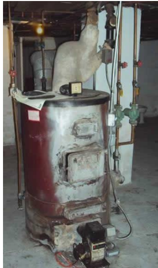
Examples of asbestos insulation wrapping boilers and associated pipe insulation encapsulation.
