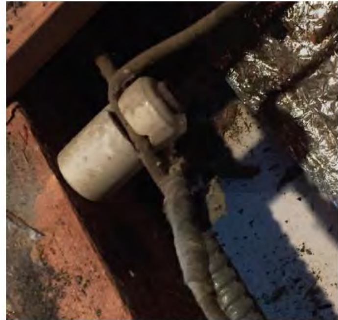
Close-up of typical ceramic "knob" circa 1925.
